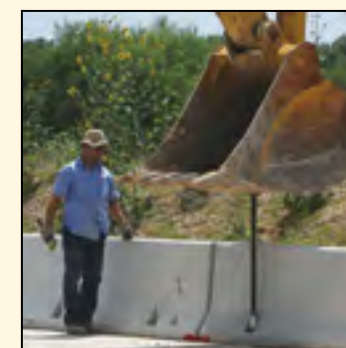
Pins installed - 3 minutes each
