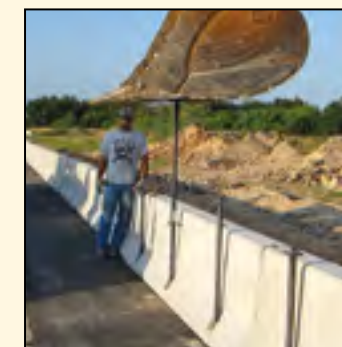
Threaded removable pin extension used for installation & removal
