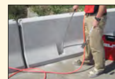
Cleaning hole with air and brushing
