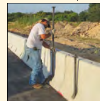
Threaded removable pin extension used for installation & removal
